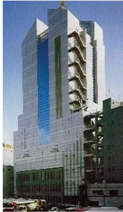
(b) Completed Building
