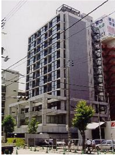
(a) Overall view of building
