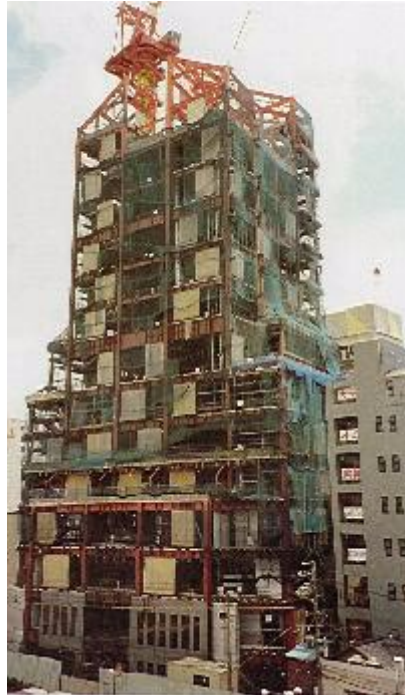
(a) During Construction
